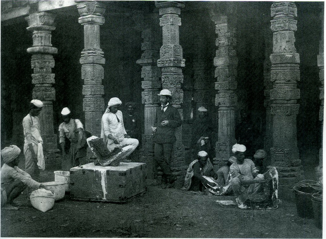
10. Charles Shepherd. Casting operations in process, under the supervision of H. H. Cole, at the Quwwat-ul-Islam mosque complex, Delhi, c. 1870. Albumen print. Courtesy of The Canadian Centre for Architecture (CCA), Montreal. Reproduced from Pelizzari, Traces of India .
