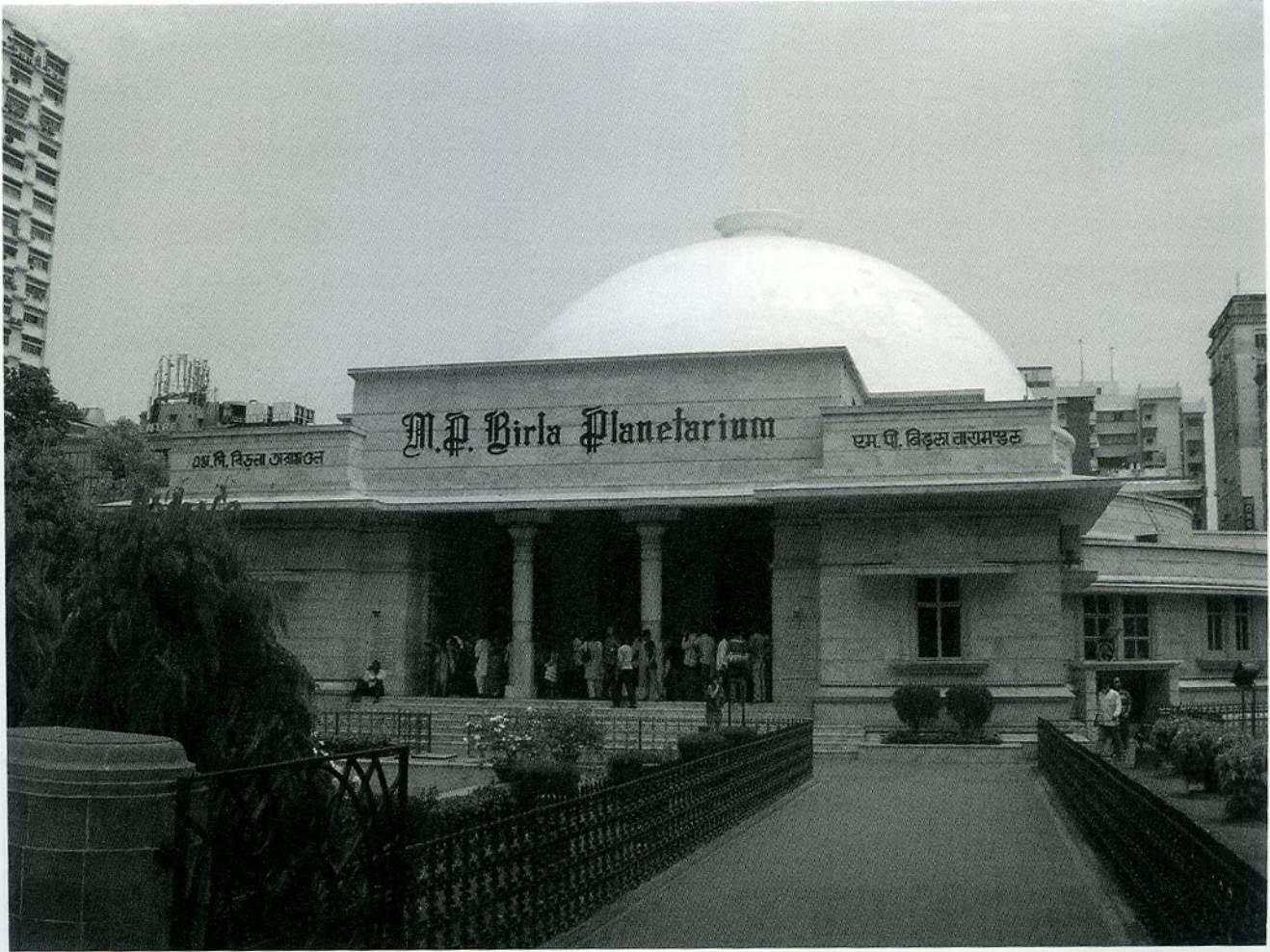
20. and 21. Hemispherical dome and balustrade railing of the M. P. Birla Planetarium, Calcutta, the oldest in India, established in 1962.
